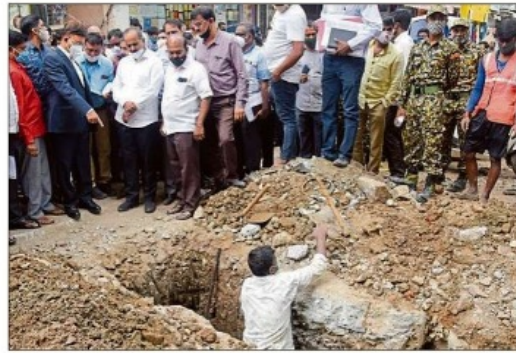
BBMP Administrator Gaurav Gupta, MP P C Mohan and BBMP officials inspect civic works on Wednesday. DH PHOTO/S K DINESH
