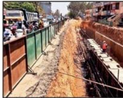
INFRA HURDLES: Traffic problems during the Kundalahalli underpass work prompted BBMP to look for an alternative technique
