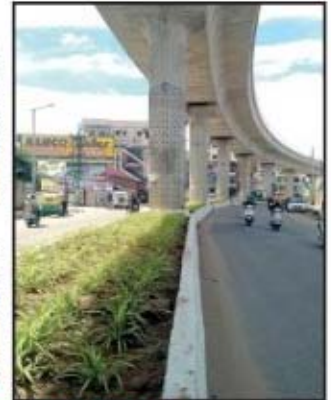
NEW ADDITION: The Kanakapura Road (Yelachenahalli-Anjanapura) section may open by December 15
